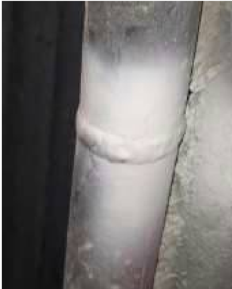
Figure 5 DP testing of PSH DMW joints
