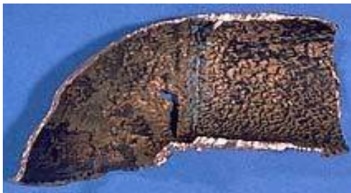
Erosion-Corrosion Damage in pipe line
