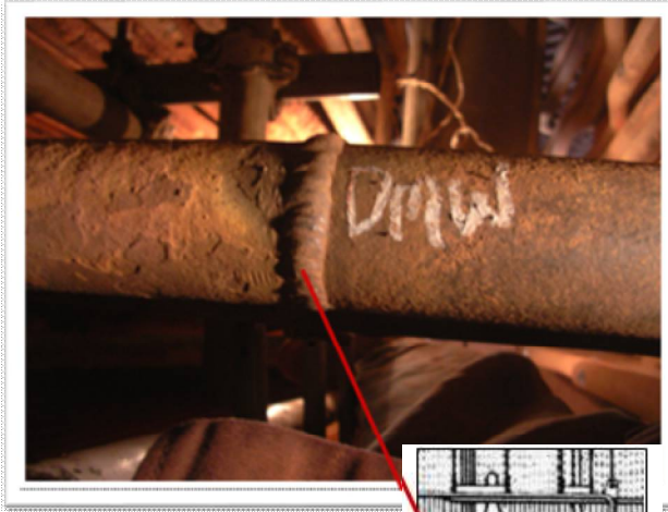
Damage to DMW joint
