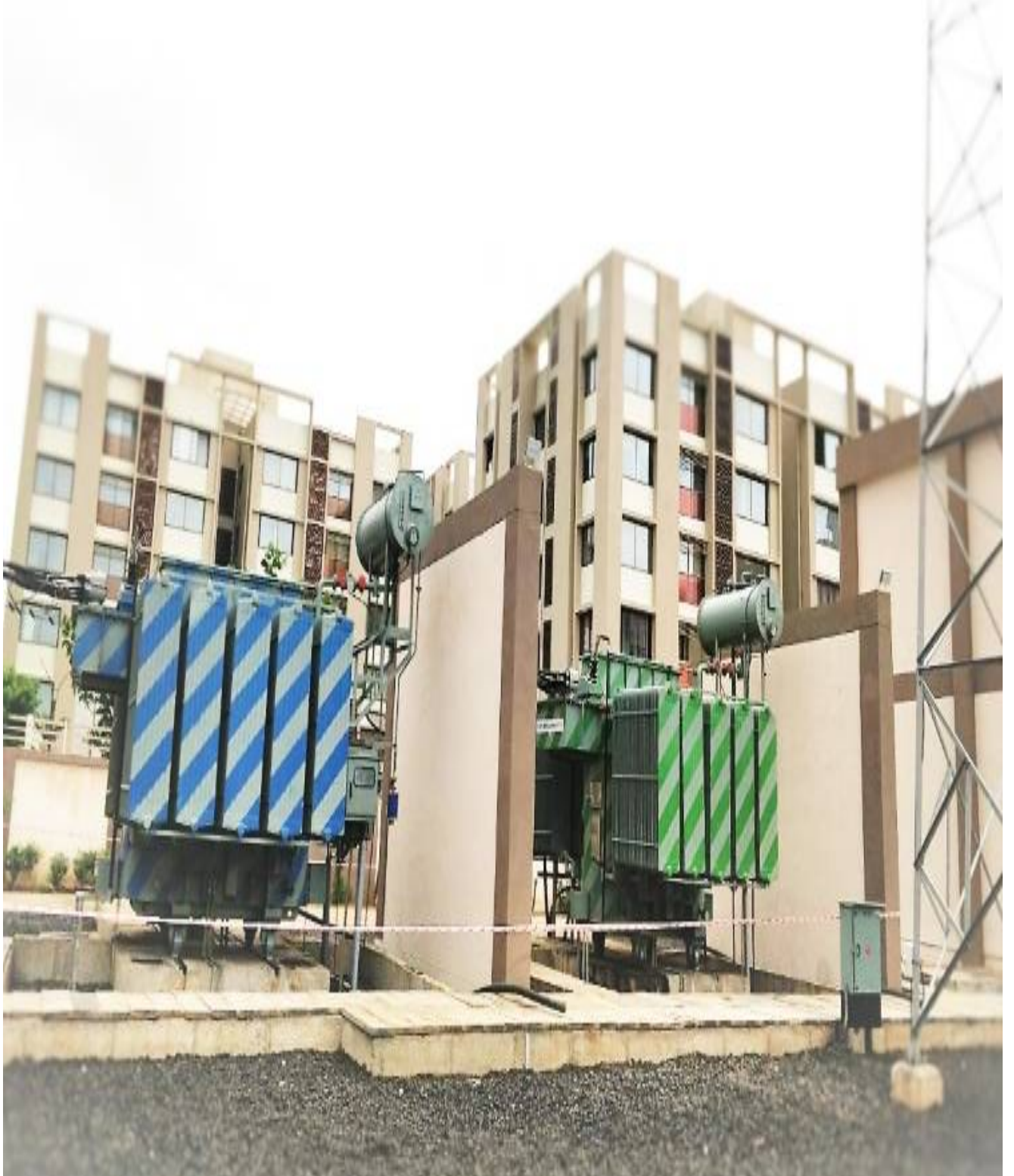
Actual site image of Atlanta make Natural Ester oil filled transformer
