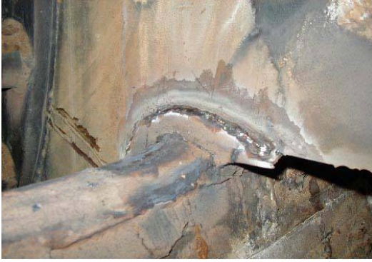
Fan Liner Protected with Chrome Carbide weld overlay after 4 months service.
