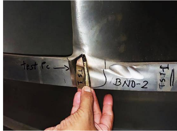
Fig.4: Francis Turbine Blade no.2 Damage due to cracking & erosion
